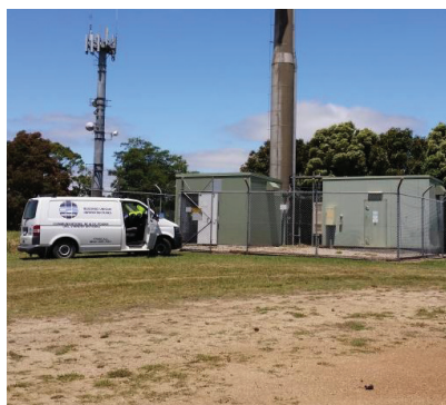
Installation onsite at Camp Hill, Victoria
