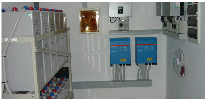
New batteries installed
