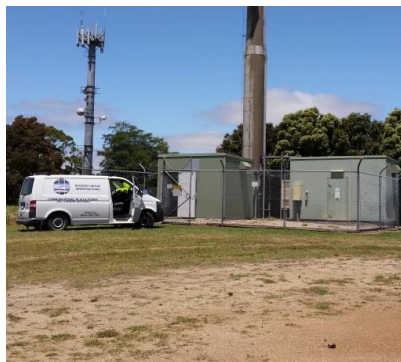
Installation onsite at Camp Hill, Victoria
